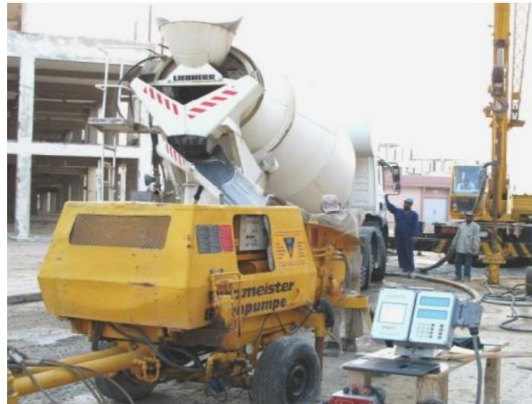
Figure 2: Delivery of cavity filling mix
