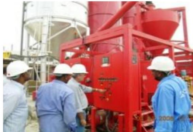
Figure 7: Insite slurry preparation
